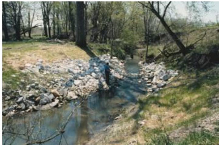
**Figure 11.** Pool and riffle structure in Blue Creek watershed
