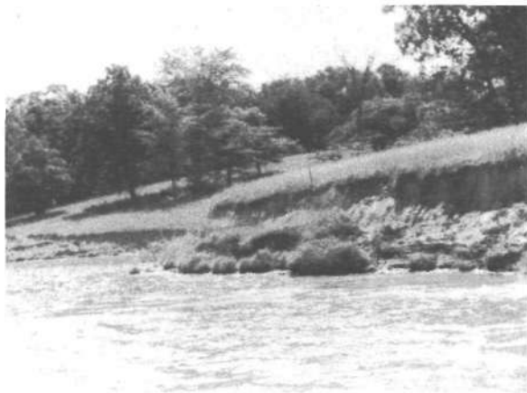
FIG. 5. SHORELINE EROSION, LAKE BRACKEN.
