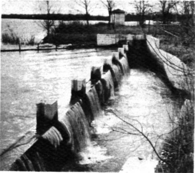
FIG. 2. WEST FRANKFORT RESERVOIR SPILLWAY - 1951.
