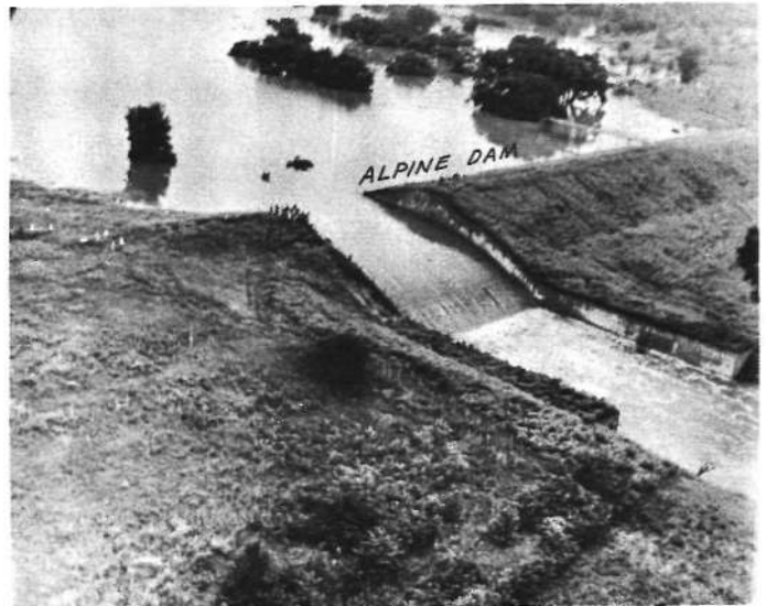
FIG. 12. VIEW OF ALPINE DAM AND FLOOD CONTROL RESERVOIR ON KEITH CREEK
