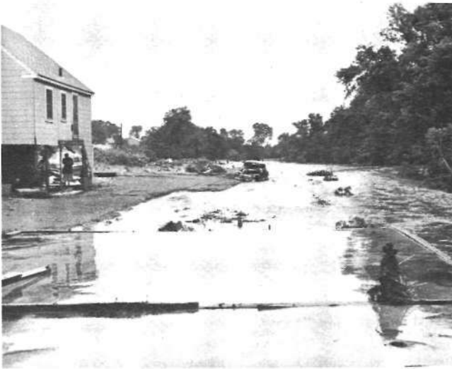
FIG. 1. PELLEY ROAD CREEK. IN FOREGROUND FOUNDATION OF HOME THAT WAS SWEEP AWAY
