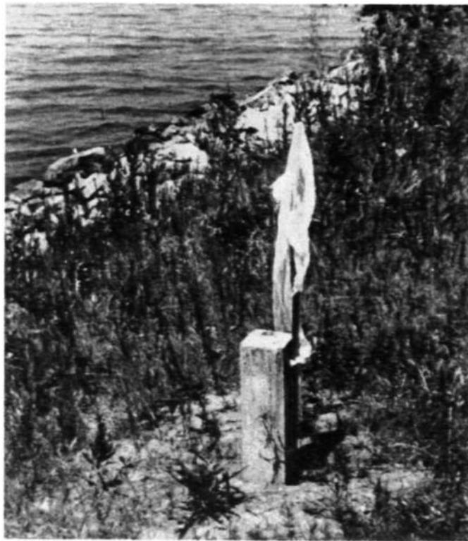
Figure 4. Concrete Post Used to Mark Survey Stations.
