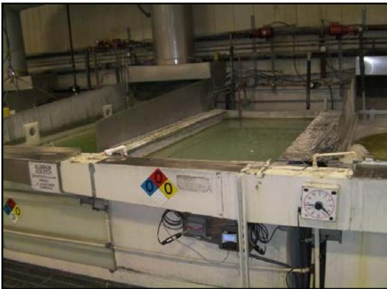
**Figure 1: Rinse Tank 2 with conductivity controller and solenoid bypass switch mounted under overhang**
