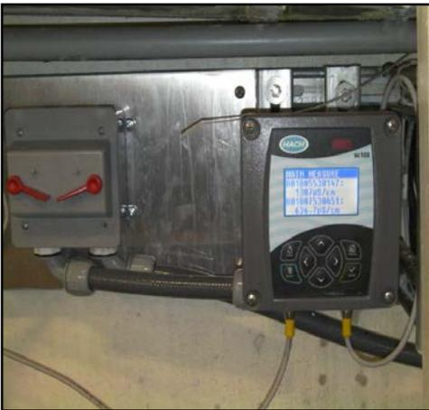
**Figure 2: Conductivity controller and solenoid bypass switches**
