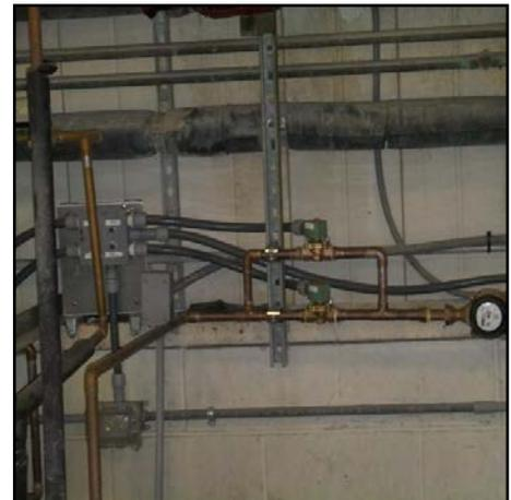
**Figure 3: Solenoid & meter installed in water supply lines**
