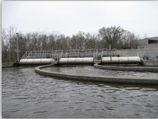
**Figure 1 : Oxidation ditch with aerators in background**
