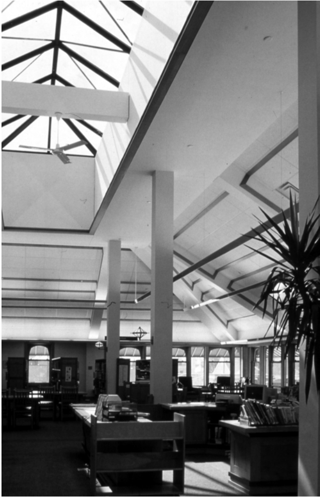
Figure 1. This library has a beautiful skylight, but as the sun crosses the sky during the day, a band of intense direct glare crosses the library. When the light falls on the service desk at midday, it's a terrible place to work, and the staff computers there are unusable. Source: Fred Schlipf.
