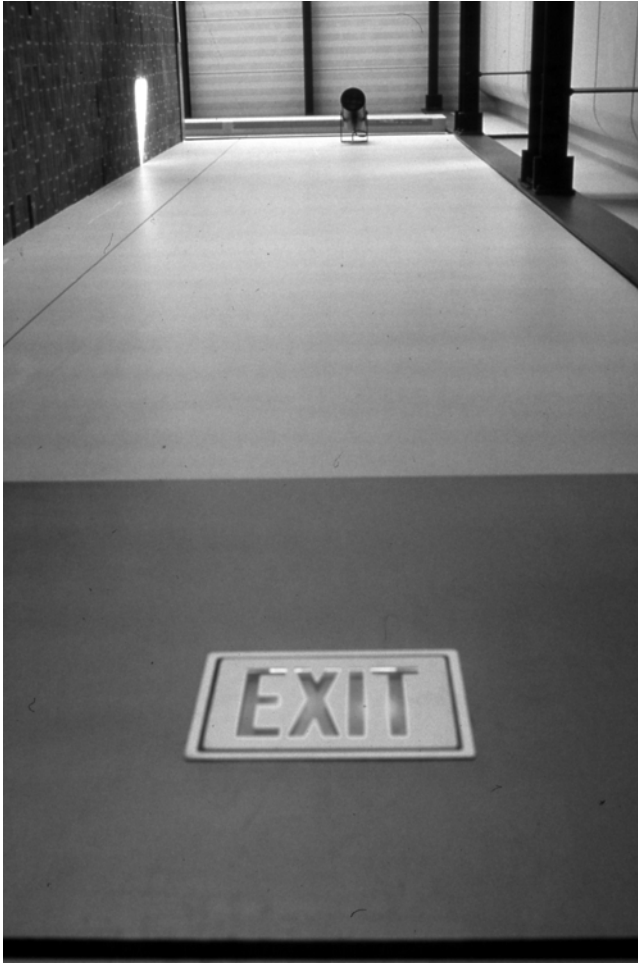
Figure 4. The burned-out lamp in this light fixture at the University of Illinois has been changed only once because the university couldn't afford to build another scaffold to change it again. Source: Fred Schlipf.
