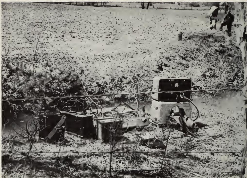
Fig. 4. - Portable seismograph equipment being used at Station 64.
