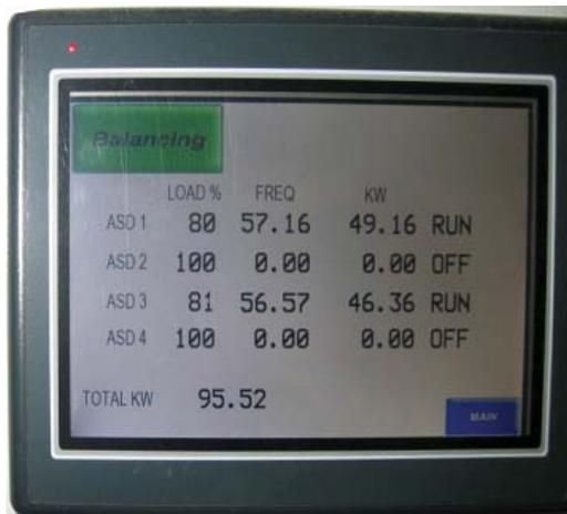
Figure 2: VFD Control Panel showing electricity consumption and performance after installation
