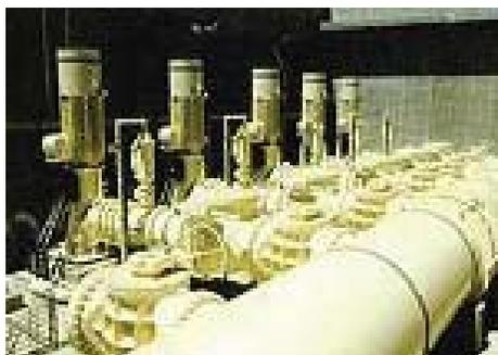
Figure 4: Common header application
