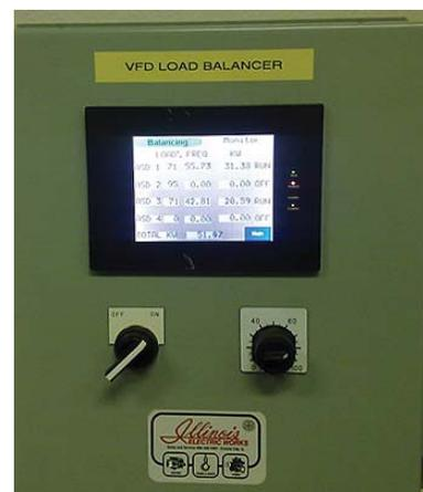
Figure 5: Load balancer
