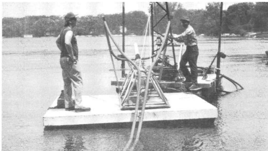
*Survey staff get ready to install an aeration device into Lake Catherine in the Fox Chain of Lakes, site of successful experiments to restore lake water quality by mechanical mixing of oxygen-poor bottom water with oxygen-rich surface water, combined with chemical treatments. These methods, developed in the late 1970's, are proving useful in restoring water quality in water supply lakes and reservoirs in other Illinois communities.*
