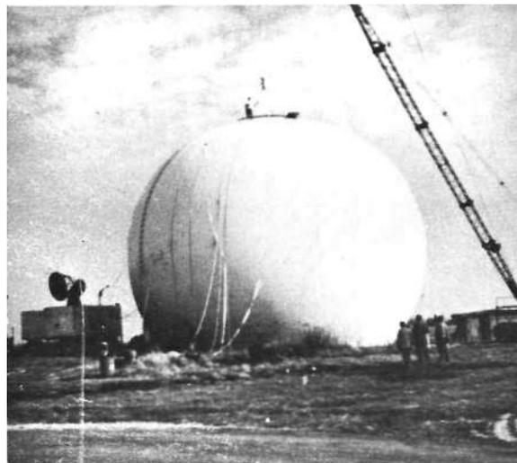
*Figure 1. Sequence of photographs showing the erection of the radome over the 10am antenna in Illinois*
