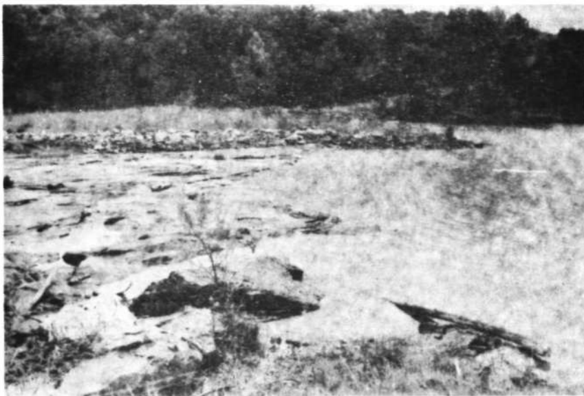
Figure 7. Spillway for Little Cedar Lake
