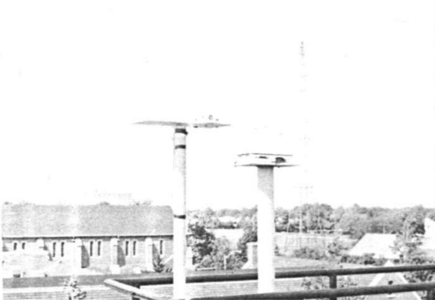
Figure 3. Champaign site, August 1981. Eppley 8-48 pyranometer on left-hand stand and actinograph on right-hand stand. View from top of penthouse on east-end of Water Resources Building, looking NE.
