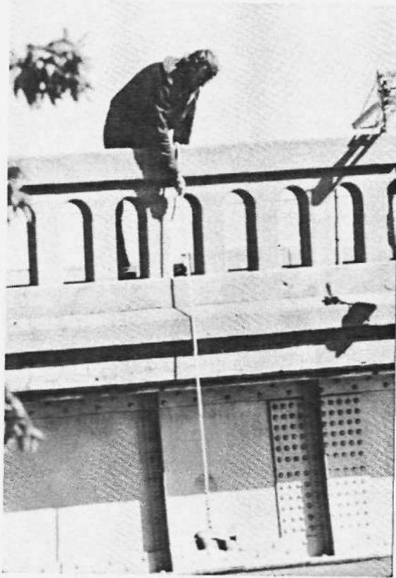
Figure 7. Technician using a US DH-59 to collect a sample
