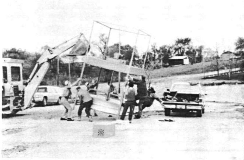
*Figure 1. Completely assembled aerator prior to its installation*
