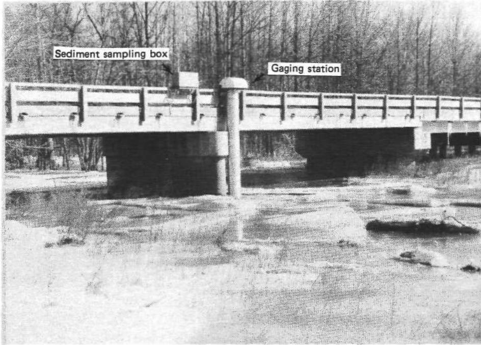
Figure 2. Gaging and sediment sampling station, Cache River at Route 146
