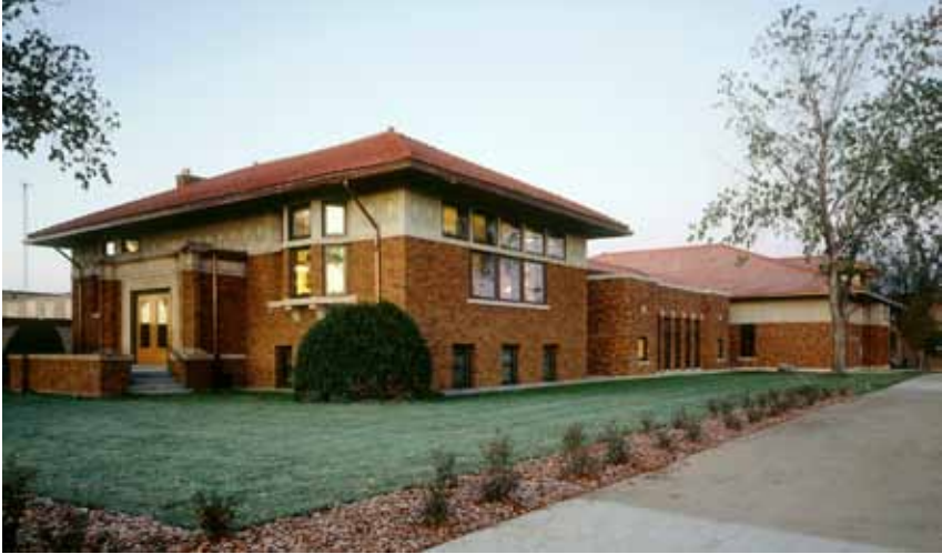
Figure 1. The Detroit Lakes, Minnesota, Public Library is one of a several libraries built using the same plans. It was expanded by MS&R (Meyer Scherer & Rockcastle), architects, Minneapolis, who designed an addition at grade level, making it possible for users to enter the building without using stairs or an elevator and improving exit control. Photograph by Lea Babcock Scherer courtesy of MS&R.
