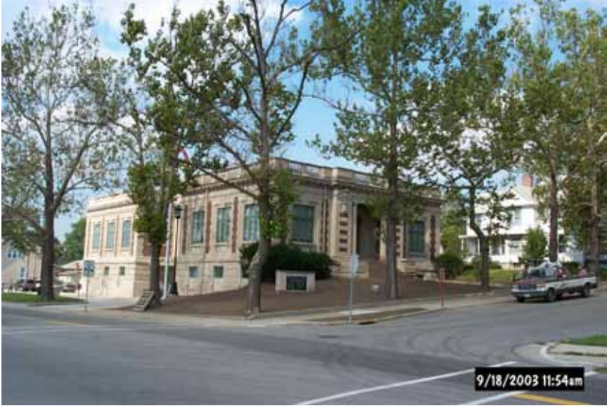
Figure 3. The LaSalle, Illinois, Public Library was located on a sloping site that allowed a new two-story addition to have a grade level entry to the basement. Photograph courtesy of apaceDesign, architects and engineers, Peoria.
