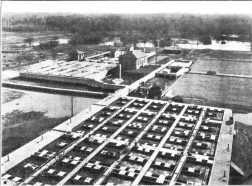
Imhoff tanks, pre-aeration plant, dosing tanks and sprinkling filters, and experimental plant. Secondary tank in background—under water because of high river.
