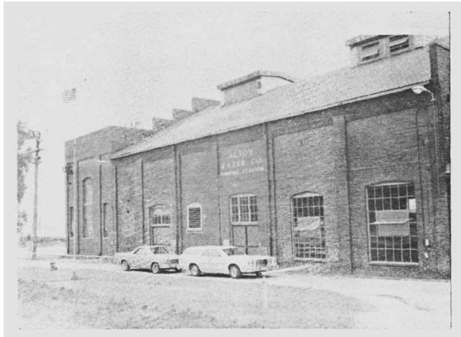
Figure 4. Main building of water plant at Alton
