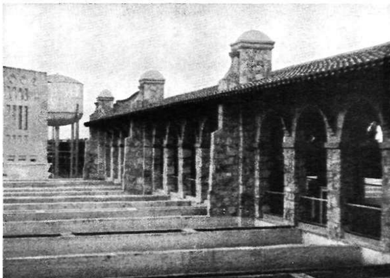
THE MILD CLIMATE AT MIAMI MAKES IT PRACTICABLE TO OMIT THE CUSTOMARY BUILDING OVER THE FILTERS OF THE SOFTENING PLANT
