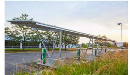
The solar project, completed in the fall of 2015, employs a total of 348 solar panel modules, capable of generating 131,800 kWh of electric power per year for the facility. This annual production is approximately 20% of the facility's electricity needs, which is approximately 8% of the company's total electricity consumption. Annually, the array is projected to reduce carbon emissions by 85.93 metric tons per year.
