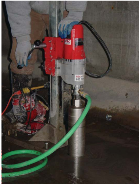
Figure 2.5. PCC drilling.
