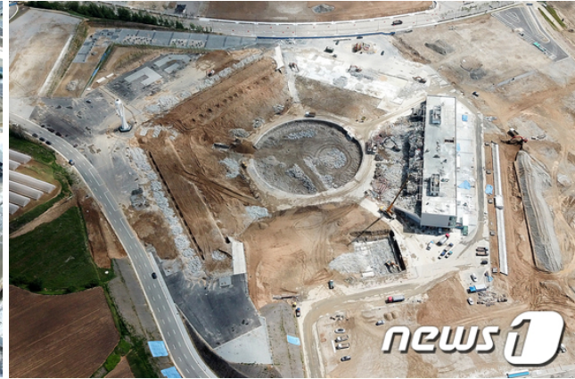
Figure 5-15. The Stadium after demolition (Kwon, 2018)
