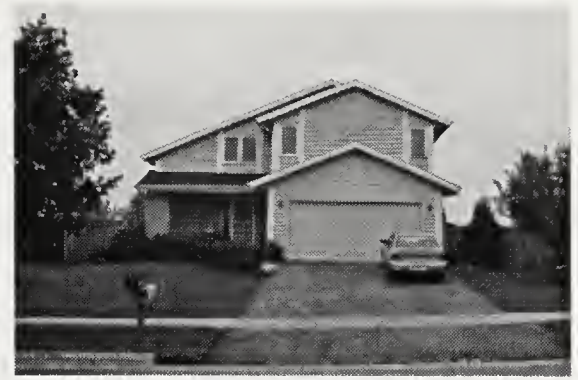
Figure 47. View from street
