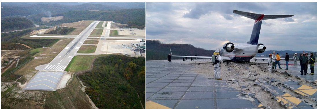
Figure 1.6. The EMAS pads (left) constructed at one end in Yeager Airport, West Virginia and (right) crushed by an aircraft in a real-world test [56].
