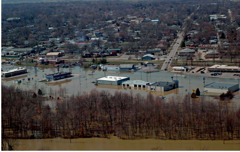
Harrisburg, Illinois did not participate in the National Flood Insurance Program and allowed development in the floodplain. The community experienced damaging flooding in March of 2008. No structures were insured against flood losses. (Photo courtesy of Harrisburg Daily Register http://www.harrisburg-il.com .)
