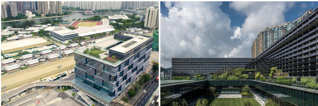
Figure 2.6: Hong Kong Jockey Club's new Communications & Technology Centre. Image source: https://www.burohappold.com
