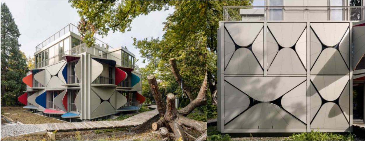
Figure 57. The Ballet Mécanique apartment block in Zürich has panels that unfold to become balconies or sun louvers. Source: https://howtospendit.ft.com/house-garden/205120-kinetic-architecture-that-s-moving-with-the-times
