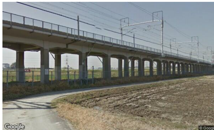
Figure 19 Google street view image of typical RC viaducts with the standard design
