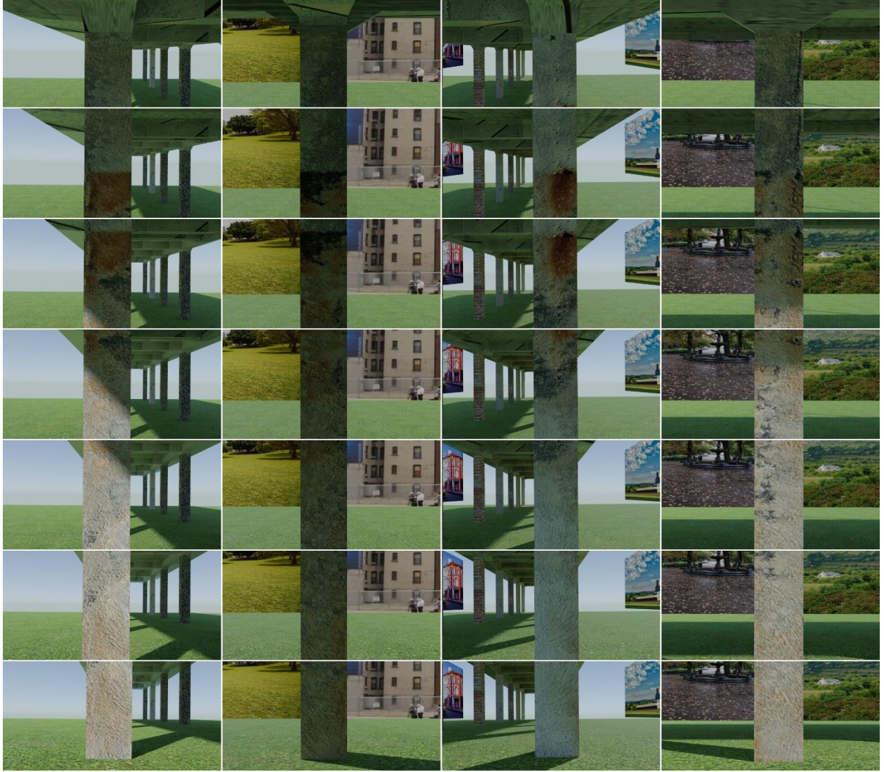
Figure 58 Images of the four faces of a column collected by the proposed UAV navigation strategy ( N_{px} = 7 , R = 0.5 ).
