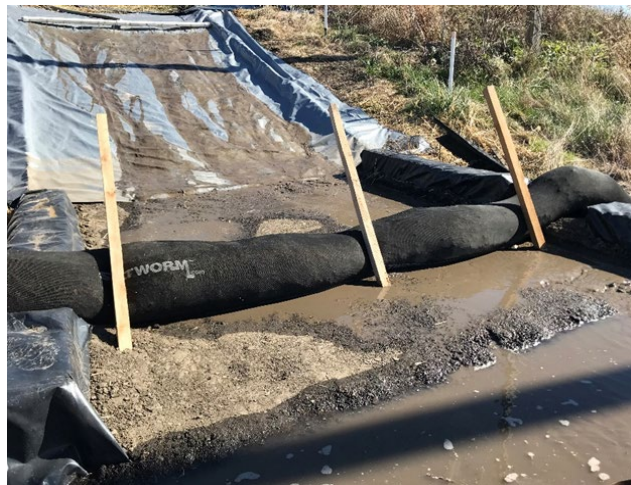
Figure 33. Photo. Percolating water under Siltworm, rather than through it.
