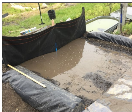
Figure 1. Photo. Silt fence (IDOT-approved fabric).
