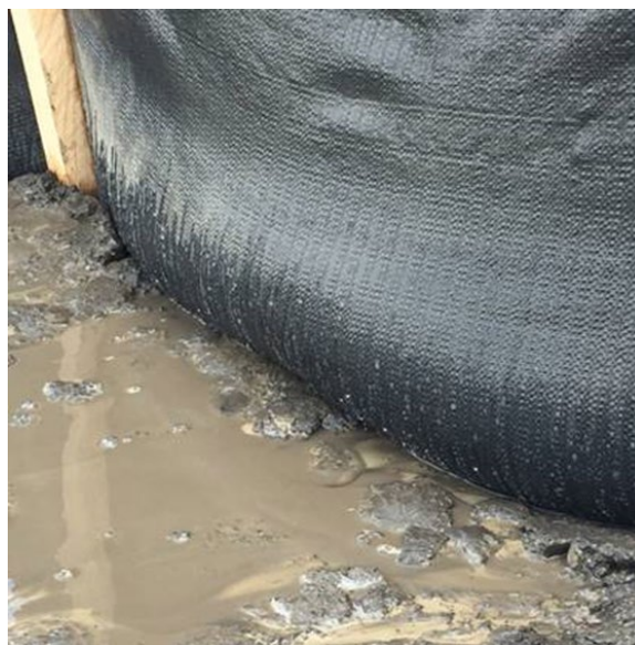
Figure 25. Photo. Clogging of silt fence during testing.
