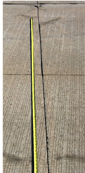
B. Distance between long. cracks at the trans. jt. (approx. 7.5-8 ft [2.3-2.4 m])
