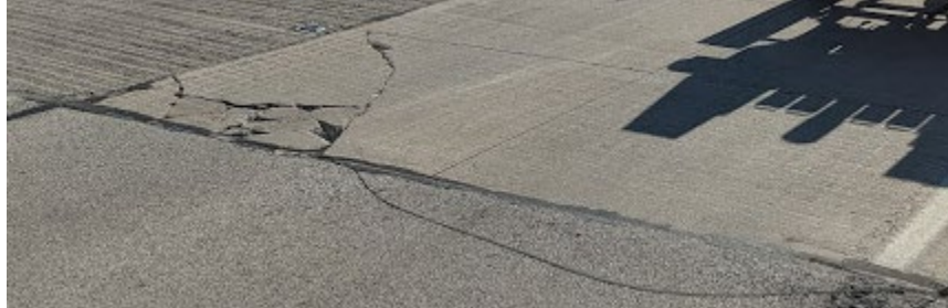
Figure 25. Photo. Distress photo of shattered slab in I-72 (72G92) eastbound.
