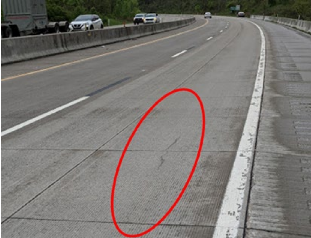
Figure 15. Photo. Pennsylvania SR-50 (eastbound) UBOL longitudinal cracking.
