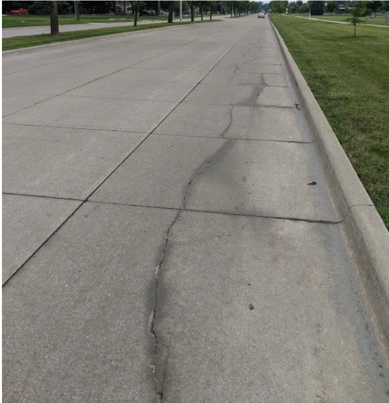
Figure 13. Photo. Hall Road (northbound) in Woodhaven, Michigan (UBOL with dense-graded interlayer).
