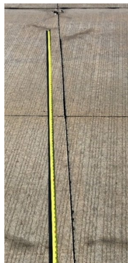
A. Longitudinal cracking in inner wheel path only B. Longitudinal cracking in both wheel paths
