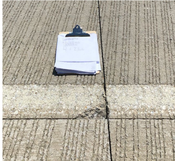
B. Grooving effect on approach joint causing corner spalling
