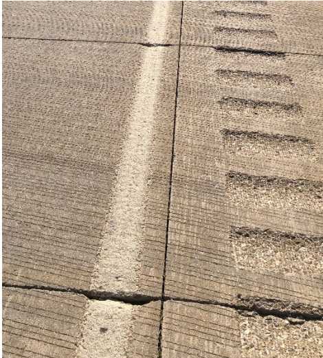
A. Grooving effect on approach joint spalling
