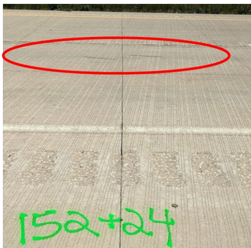
A. Longitudinal cracking in inner wheel path only B. Longitudinal cracking in both wheel paths
