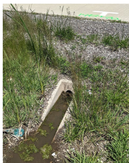
A. Longitudinal joint faulting B. Standing water in drain outlets
