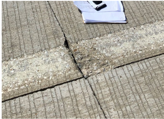
C. Grooving effect on leave joint corner spalling
