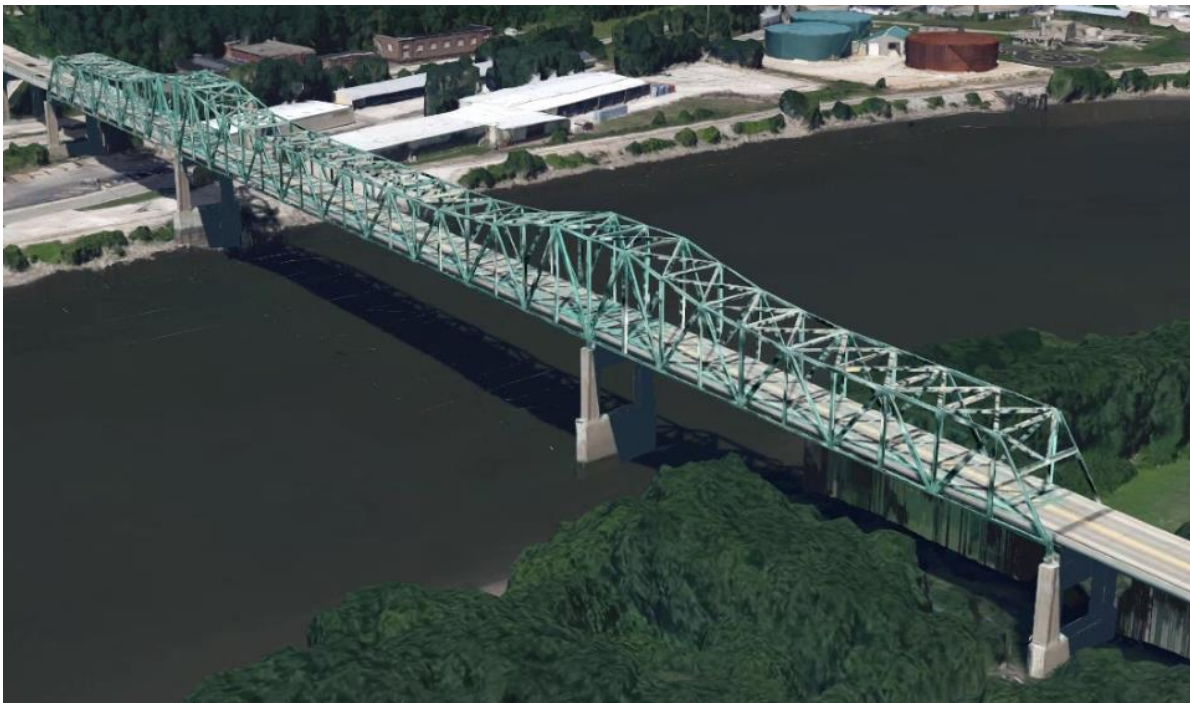
Figure 4.16. Image of the IL-251 bridge over Illinois River
