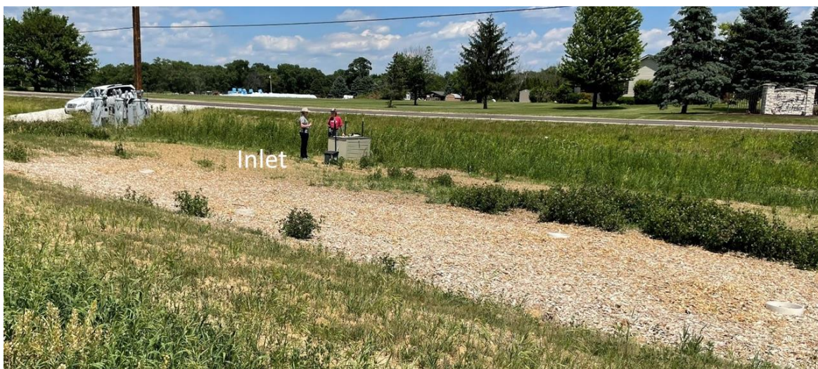
Figure 5. Bioreactor #4 - No Cover shown with the inflow control structure near the two people pictured. The outflow was to the right of the camera.
