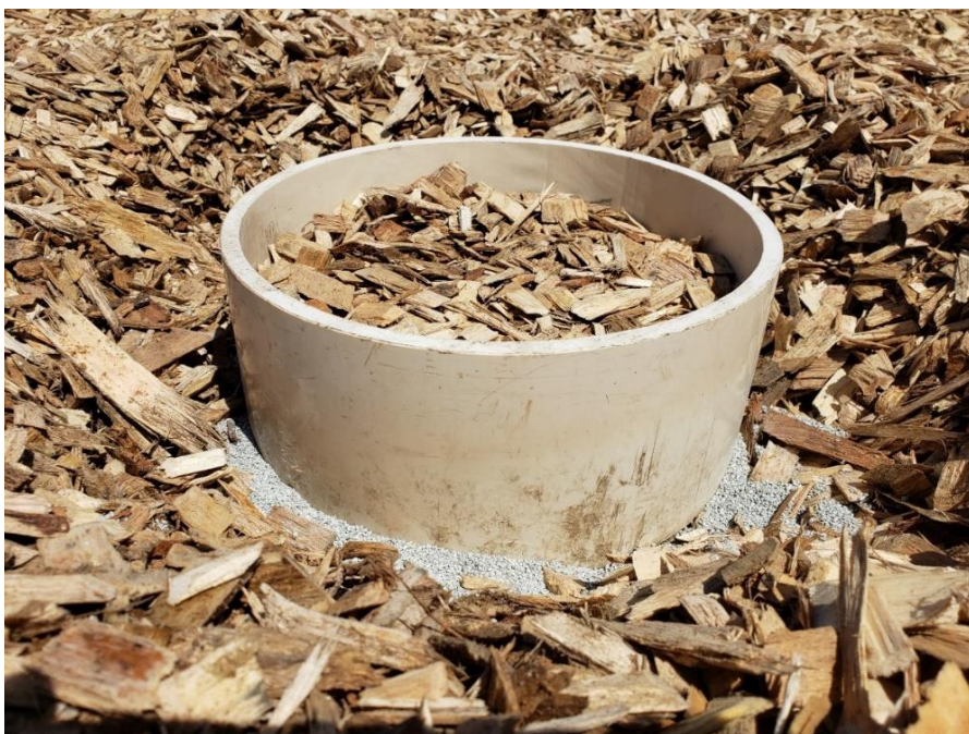
Figure 8. Chamber base installation at an uncovered site. Bentonite surrounded the edges, was soaked, and then was covered with woodchips.
