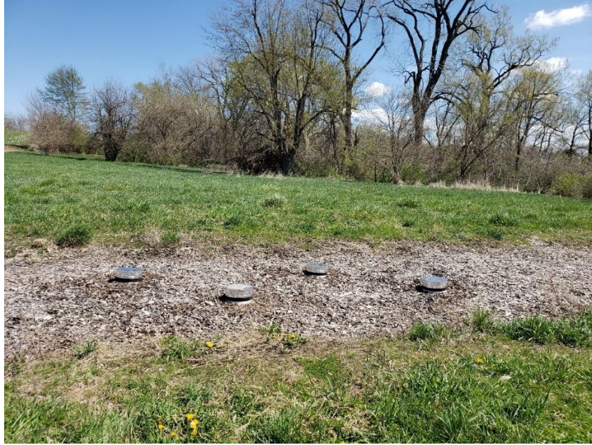
Figure 7. Bioreactor #6 - No Cover pictured from the side. The inflow control structure was to the left of the camera and the outflow was forward and to the right.
