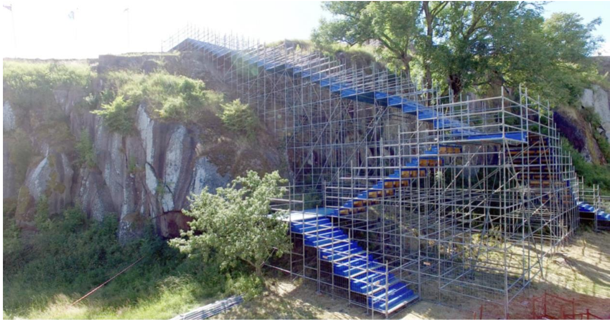
Figure 3.8: The temporary 8-story scaffolded staircase at Slottsfjellfestivalen 56
