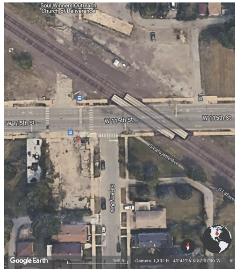
A. Chicago–115th at-grade railroad-highway crossing
