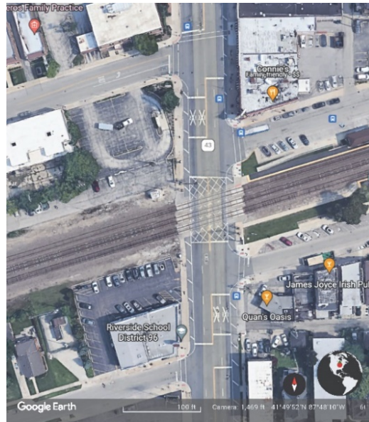
A. Riverside at-grade railroad-highway crossing
