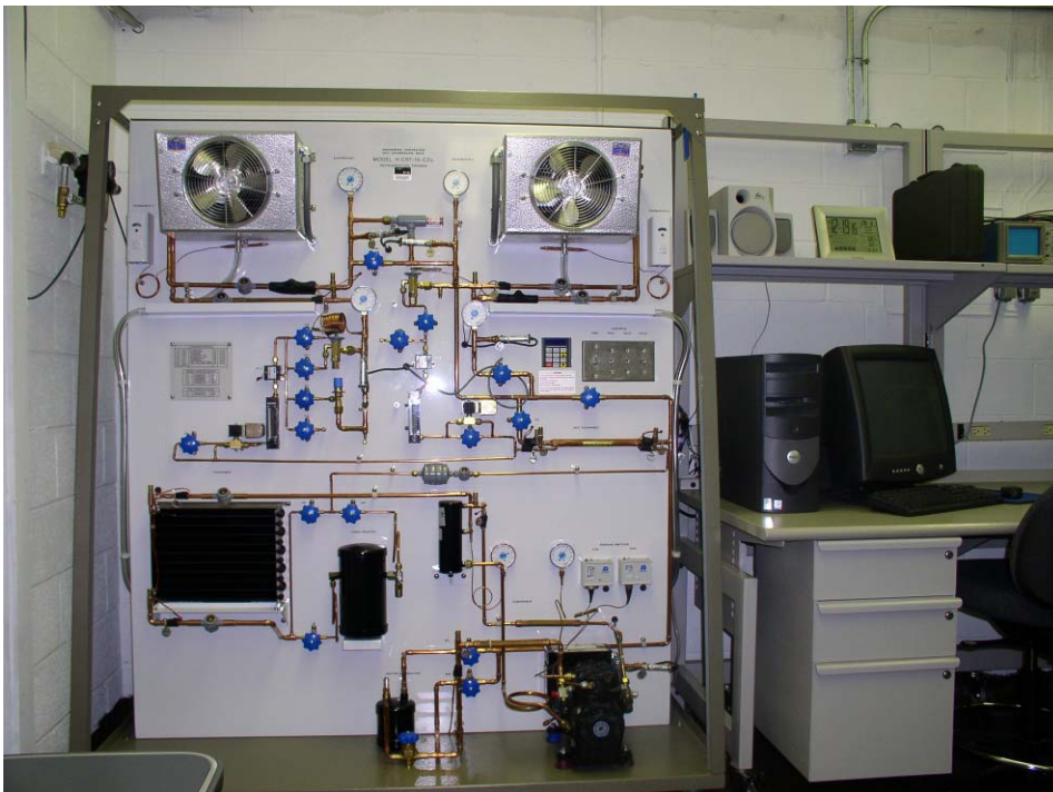
Figure 5.8 - Photo of original system
