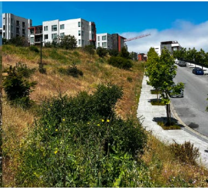
New low income housing project under construction at Hunters point.
