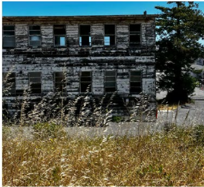
Abandoned buildings within the limits of Naval shipping yard.
