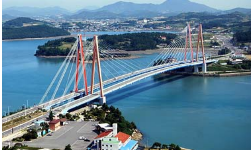
Figure 7.88 Twin spans of Jindo Bridge connecting Jindo Island with the Korean Peninsula with the newer span on the left.
