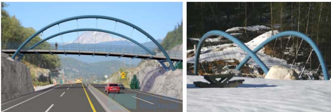
Figure 7.82 Stawamus Chief Bridge: Rendering of the completed bridge (left) and the as-built arches (right).
