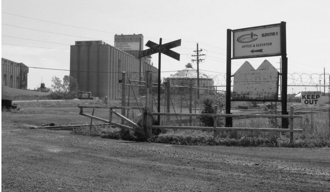
Figure 3.1: Photograph of grain silos on the Southwest portion of Lake Calumet. This today is largely vacant or has little active industry. Photograph taken by the author.
