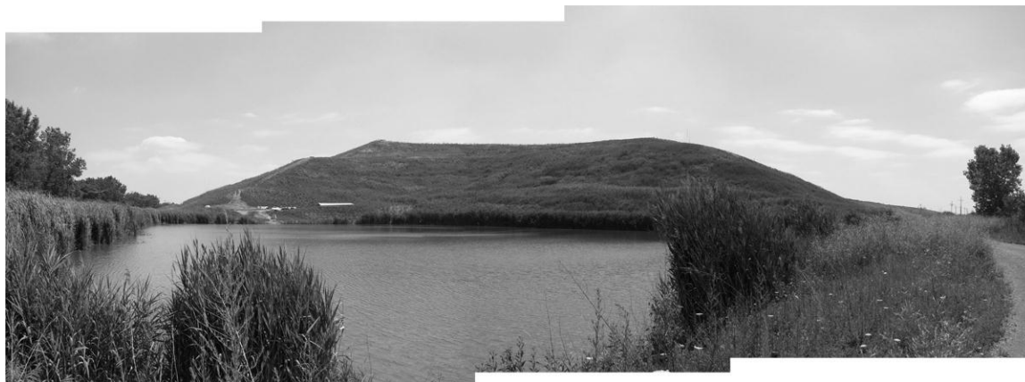
Figure 2.2: Landfill undergoing remediation in the Calumet Complex. In the foreground is a Leachate Treatment Pond. A constructed 'wetland' system largely used to de-nitrify polluted runoff. Photograph taken by the author.
