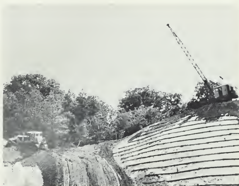
Fig. 43 — Sloping and Terracing with Dozer and Dragline
