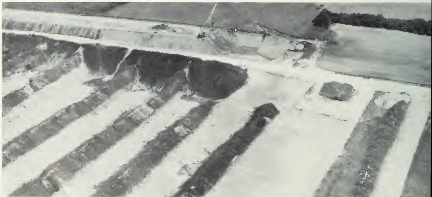
Fig. 18 — Typical Stockpiling and Excavating Patterns of the Dragline
