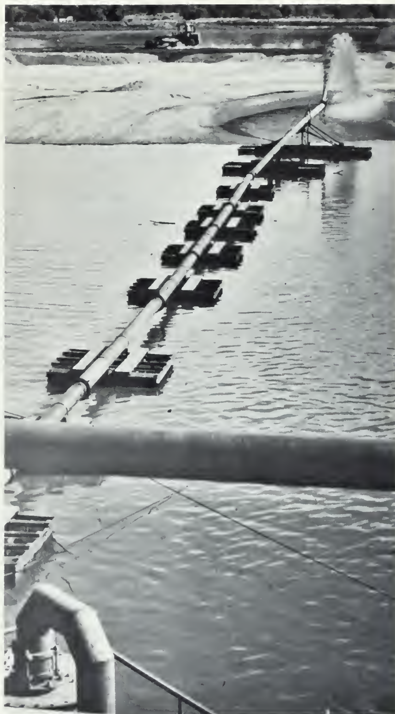
Fig. 58 — Land Forming with Waste Sand and Grading of Overburden in the Background
