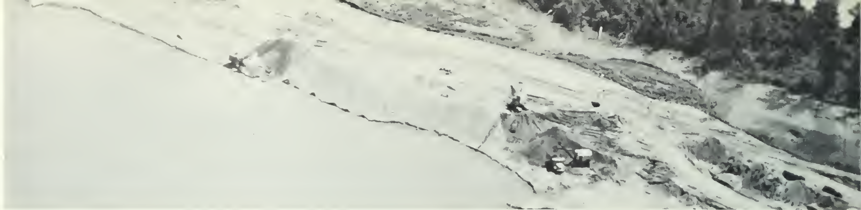
Fig. 17 — Scraper Formed Stockpile Mound
