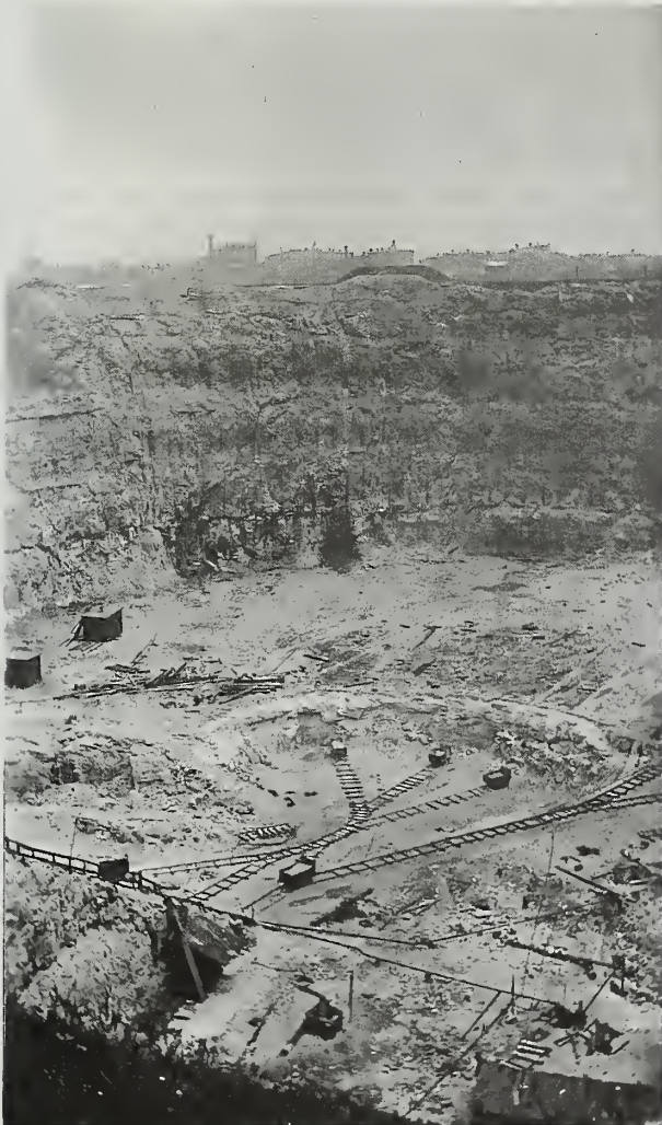
Figure 6 East wall of Stearns Lime and Stone Company quarry. Rock was loaded by hand into quarry cars, which were then pushed along tracks to the base of the incline in the lower left corner of photo. Cars were then pulled by cable up the incline to the kilns. (Photo taken in 1907 by E. F. Burchard, No. 436; Courtesy of the U. S. Geological Survey)
