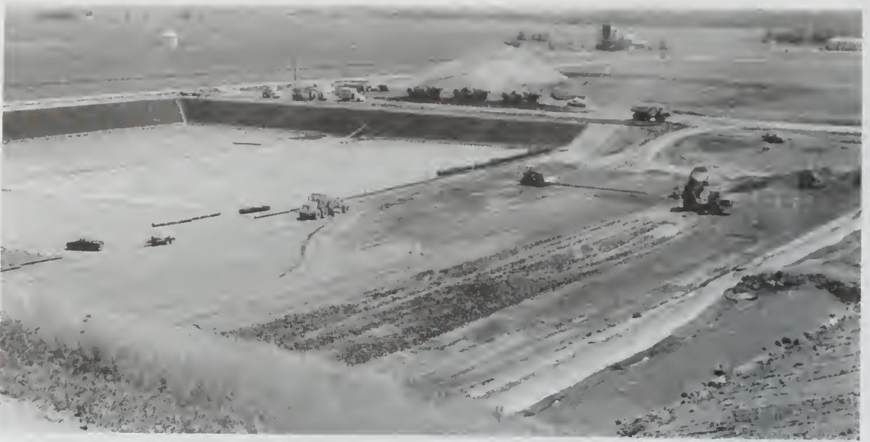
Figure 16 Landfill operation at the Envirite Corporation Landfill.
