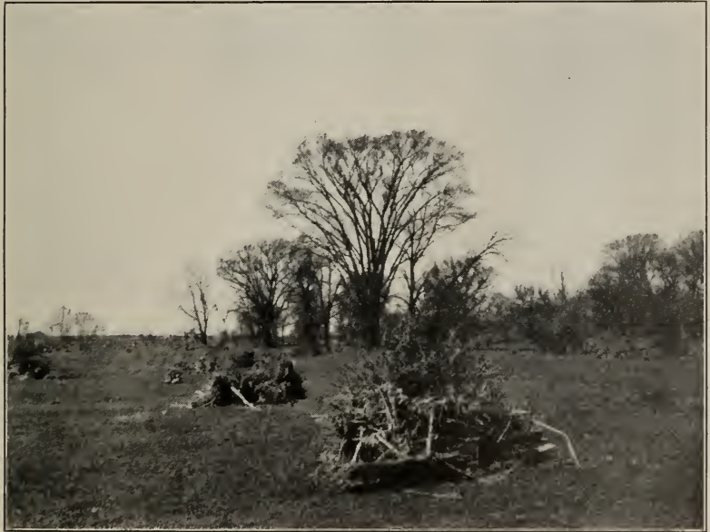
Effects of a Recent Flood on Hickory Creek.
