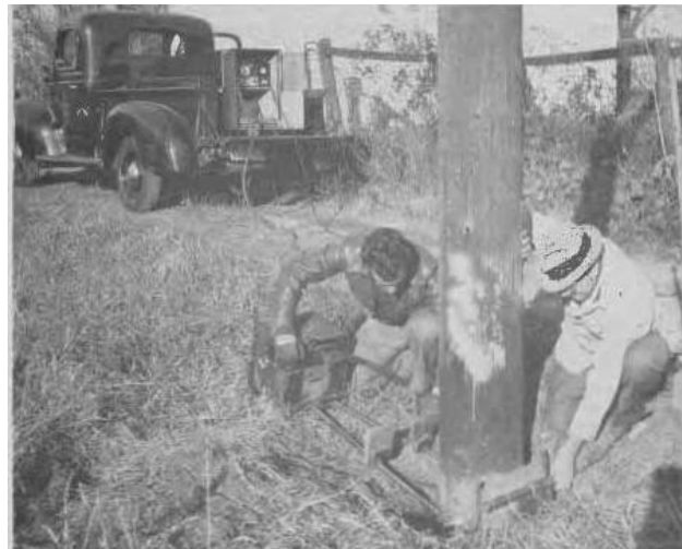
Figure 15. Radiographic setup used by Detroit Edison. Figure extracted from Stoker [40].
