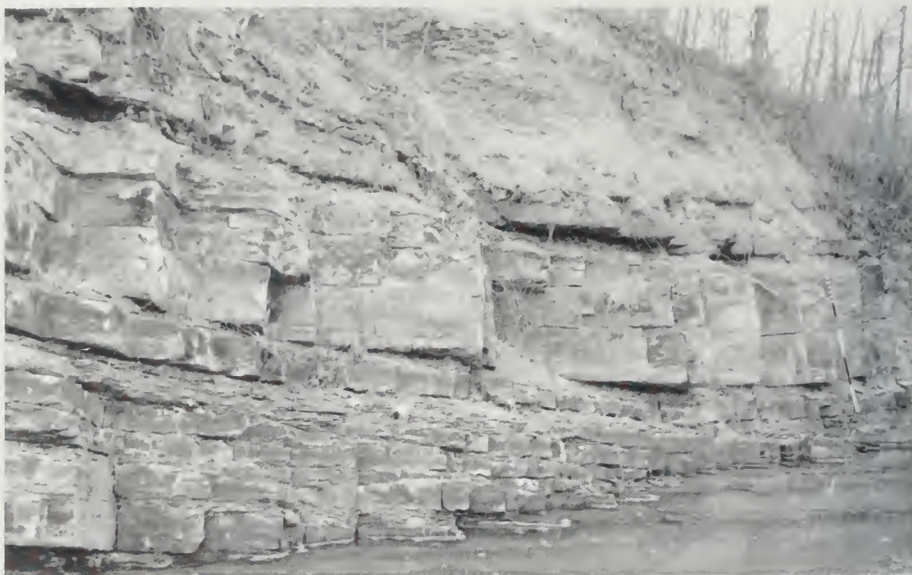
Figure 15 Basal Fort Payne Formation and upper Springville Shale in the altered area. The closely jointed, tabular-bedded rock is "calico rock" of Springville. The dark crumbly material above is ganister of the Fort Payne. Locality is in You-Be-Damned Hollow, NE SE NE, Sec. 35, T13S, R2W, Mill Creek Quadrangle.
