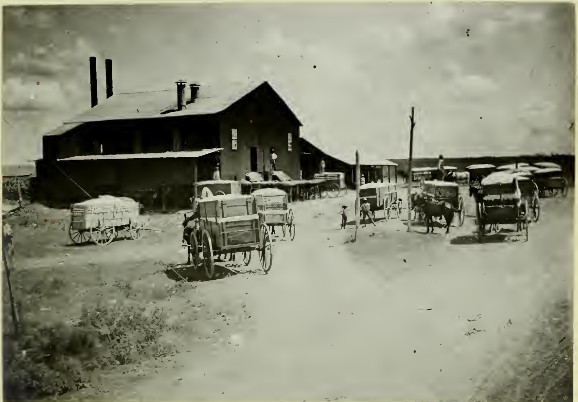
Figure 33 - Ginning Plant in Texas.
