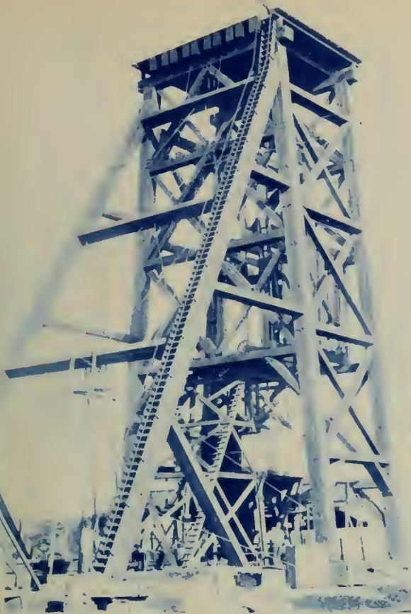
Fig. 2 - Timber Head Frame - South Africa.
