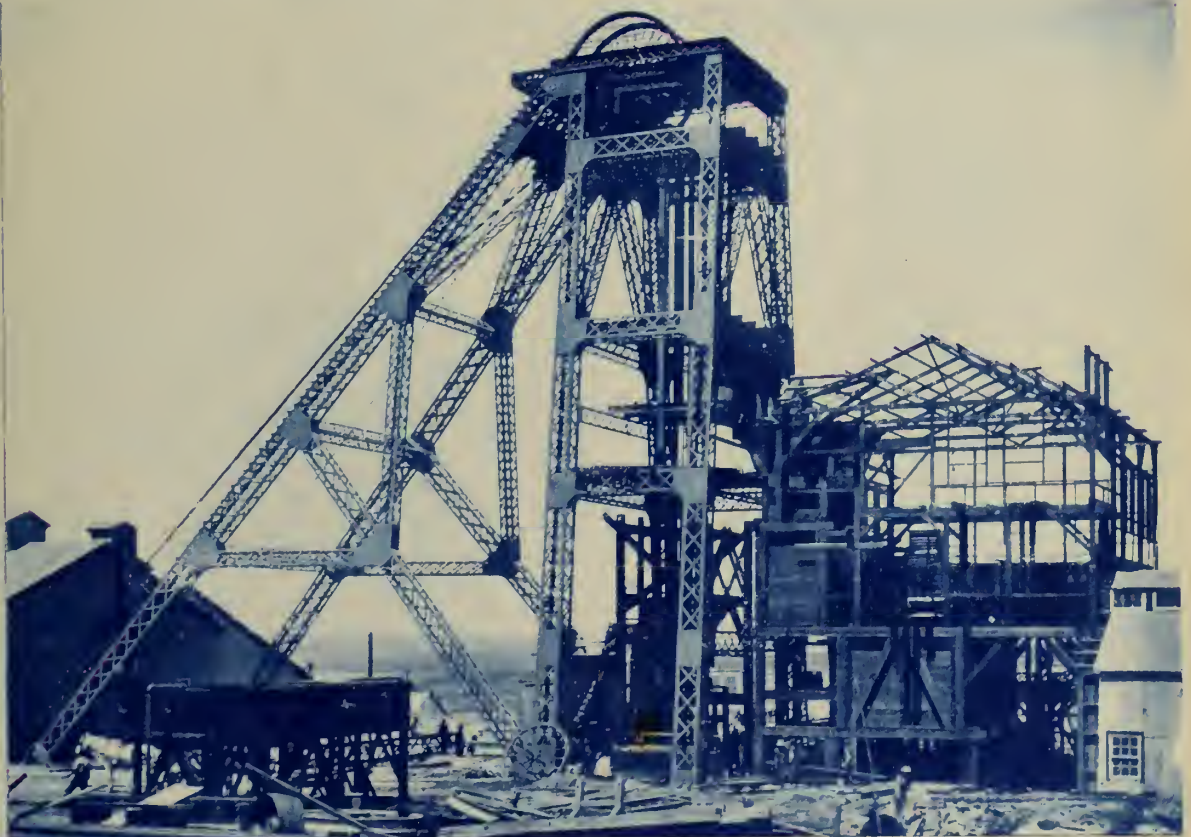
Fig. 1. Steel Head Frame - 85 ft high - Robinson Deep Mine, South Africa.
