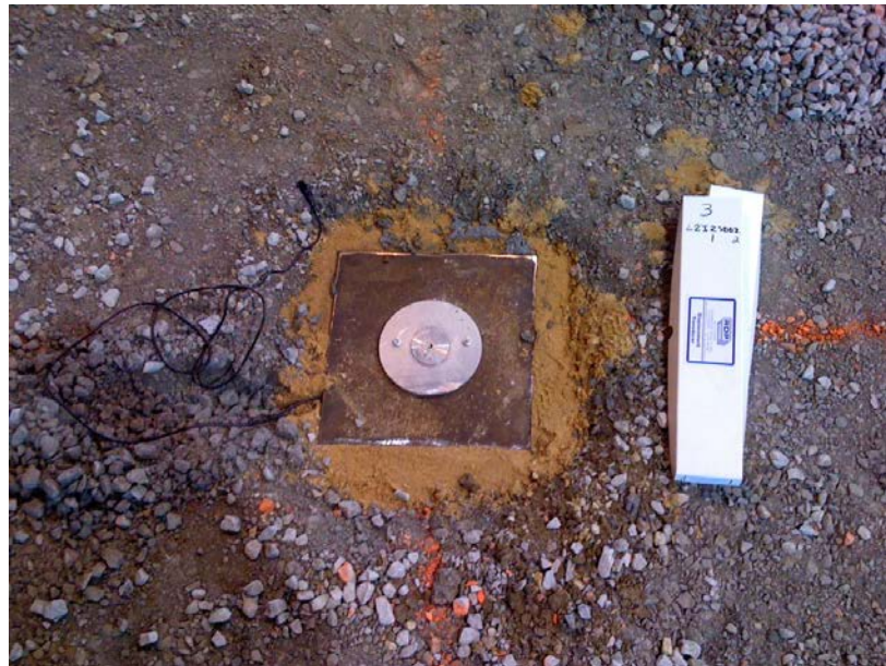
Figure 5.38 SDD after installation
