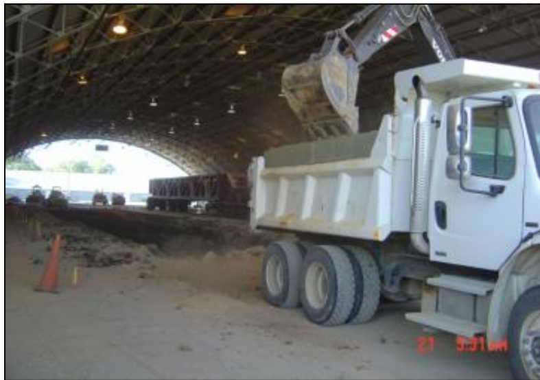
Figure 5.19 Excavation of test section
