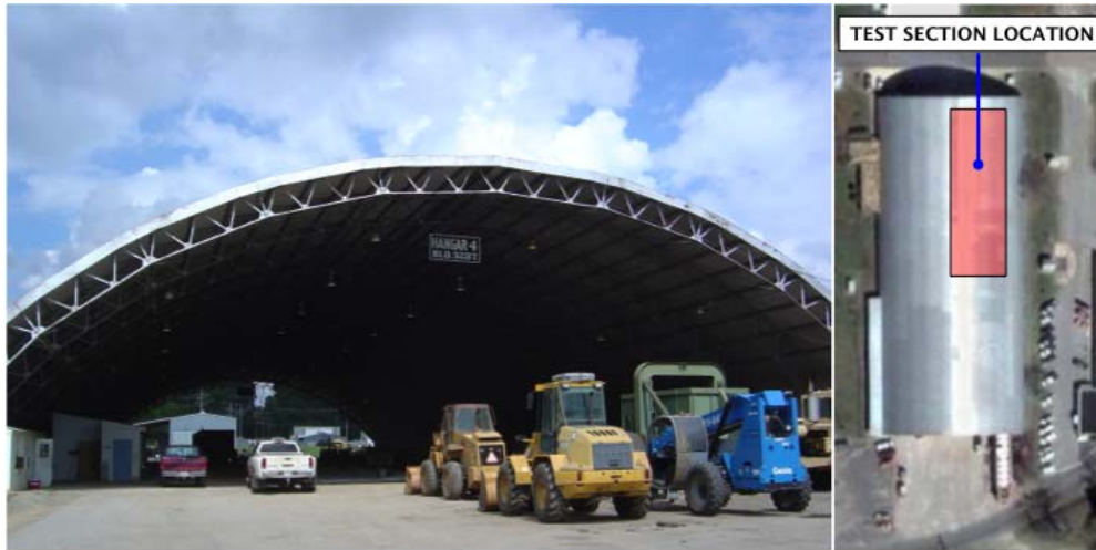
Figure 5.3 Testing facility and test sections
