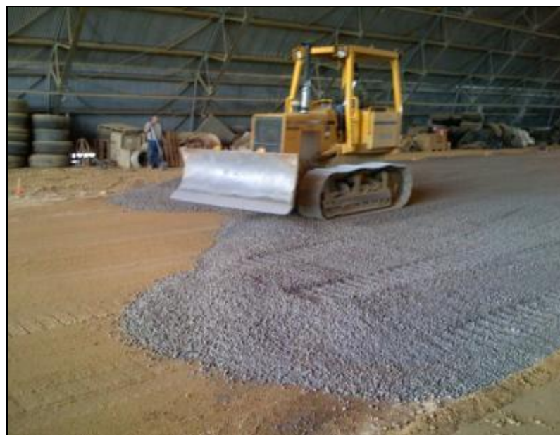
Figure 5.28 Placement of Base layer
