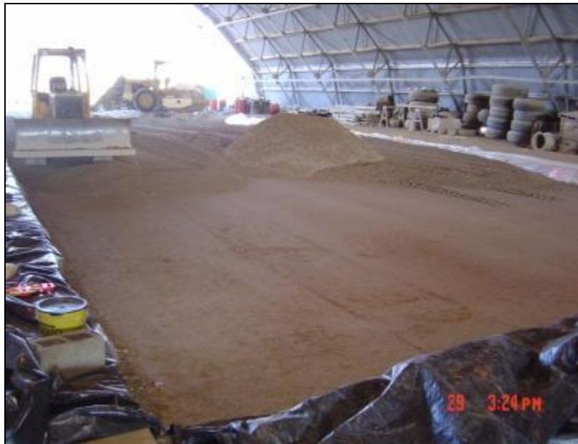
Figure 5.26 Placement of subbase layer
