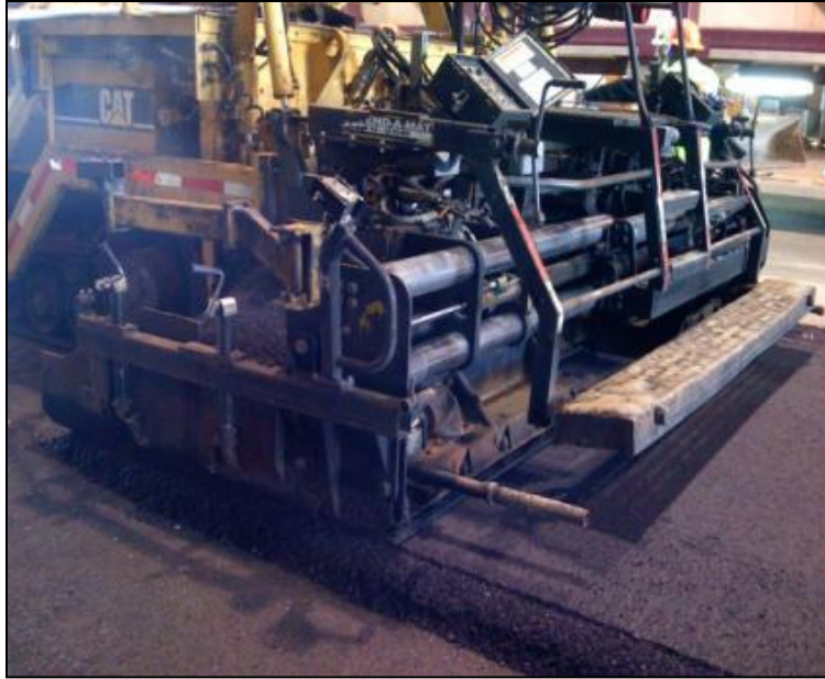
Figure 5.30 Paving operations, mat placement
