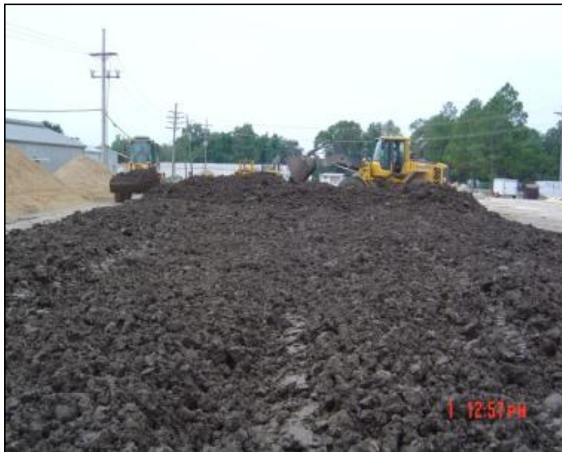
Figure 5.21 Subgrade material processing
