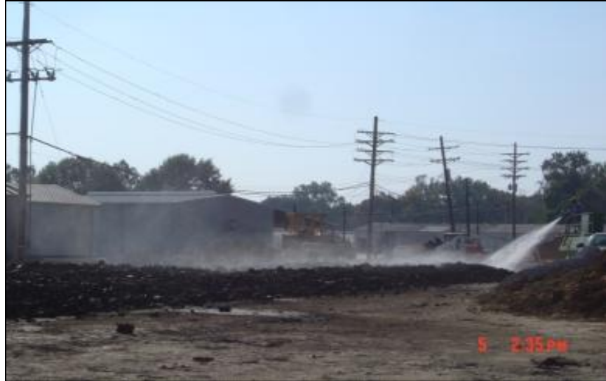
Figure 5.20 Addition of water to the subgrade material
