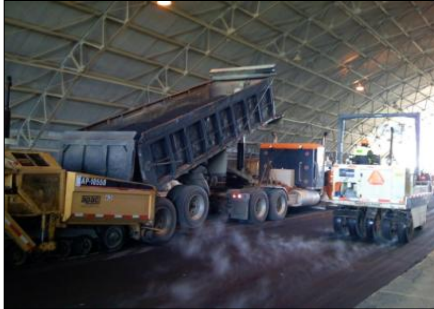
Figure 5.32 Paving operations, rubber-tire roller compaction
