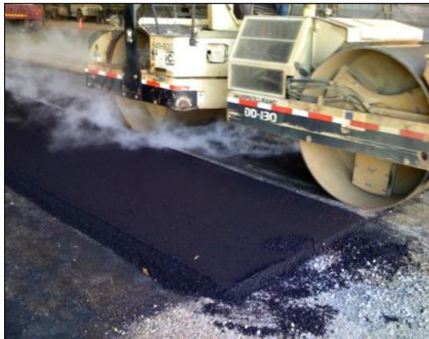
Figure 5.31 Paving operations, break-down rolling
