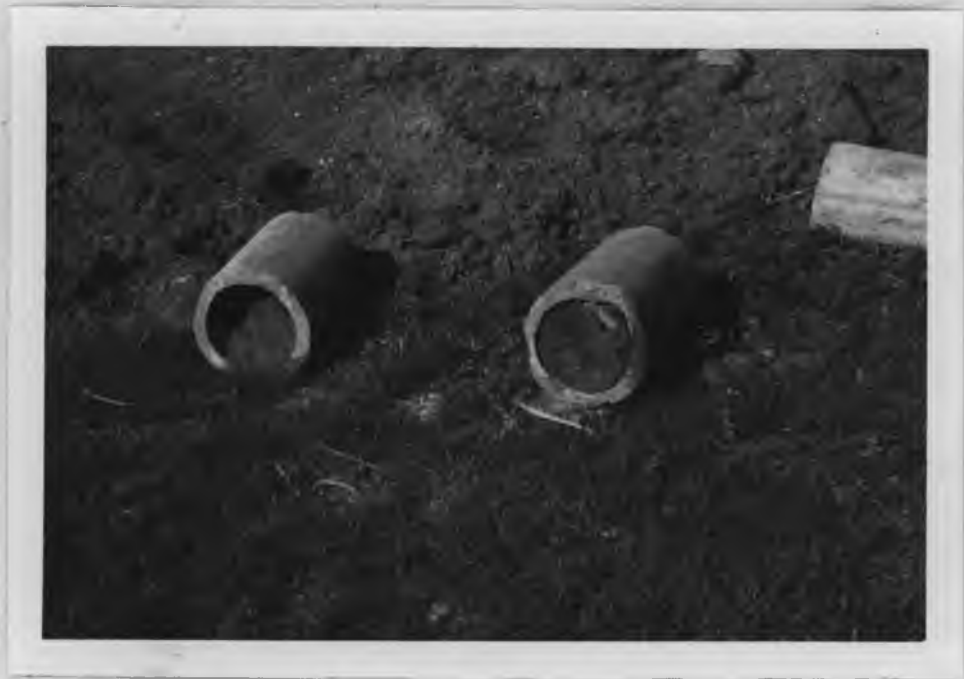
B. Silt put these tiles out of operation.
