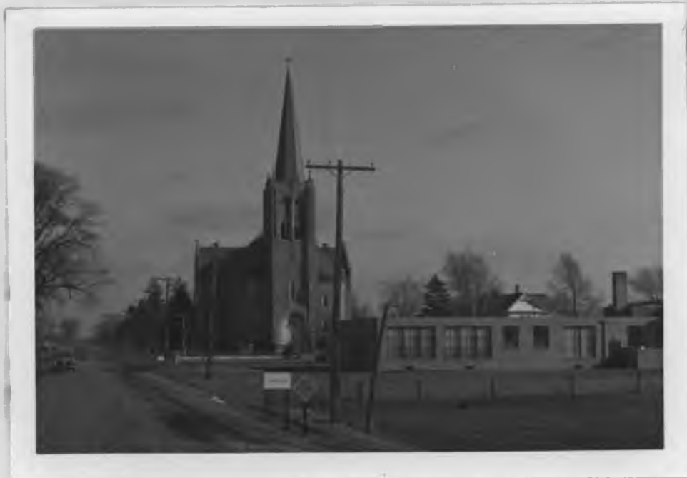
A. Front view of the church, as seen from the west.
