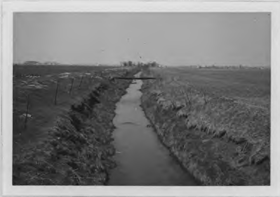
A. Main drainage ditch, Flatville Special Drainage District.
