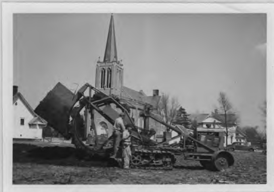
B. Laying tile on the site of the new Flatville school.
